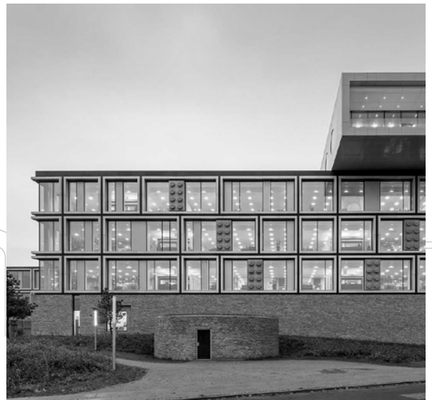
LEGO® Campus, Billund / Architect: C.F. Møller Architects
