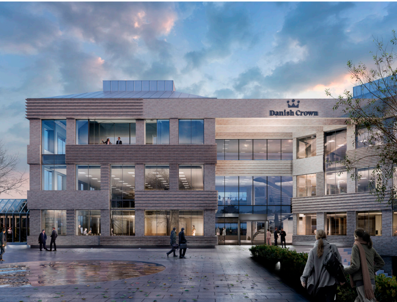
Danish Crown headquarter / Architect CEBRA architecture
