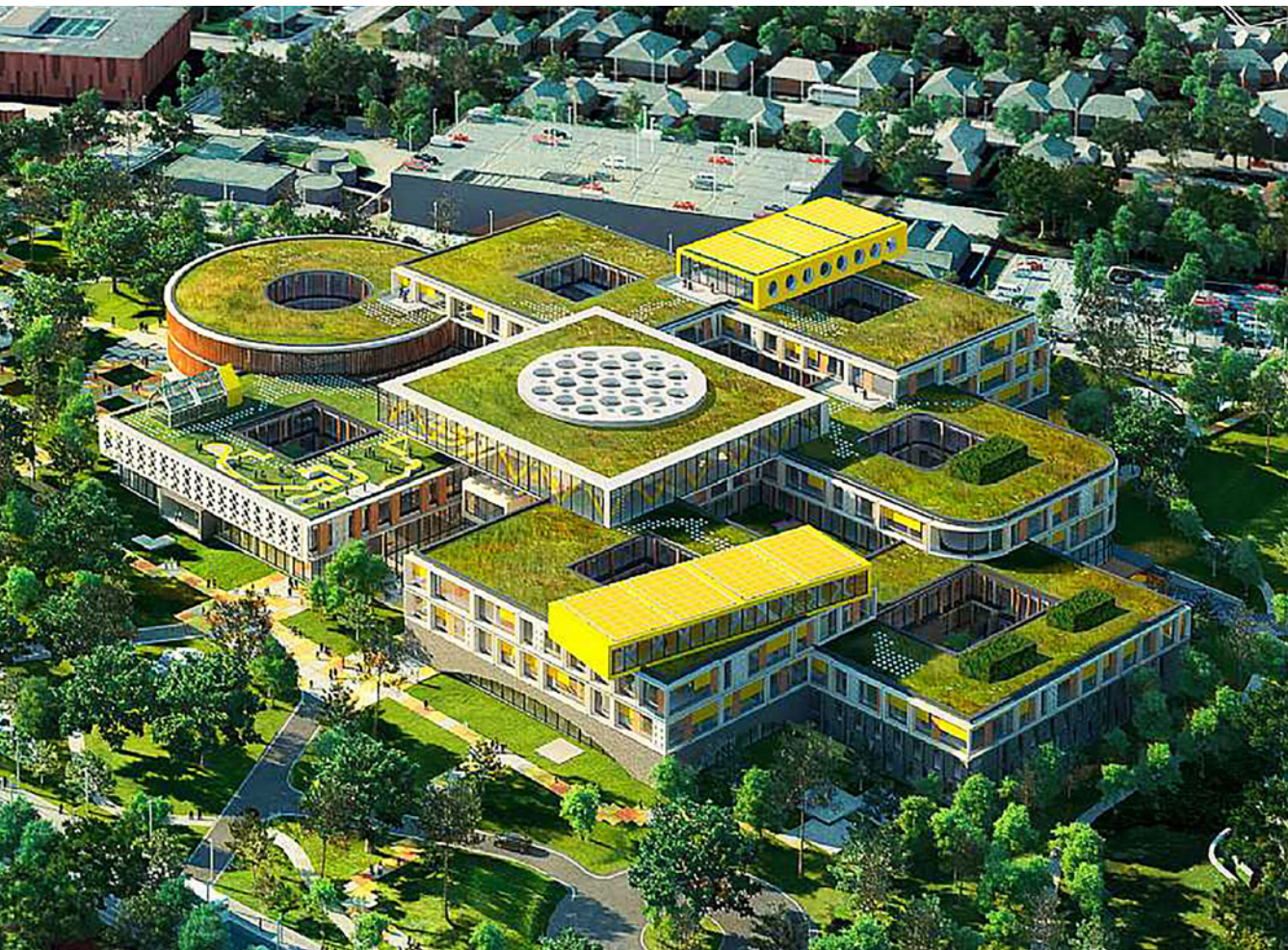
LEGO Campus, Billund Architect: C.F. Møller Architects
